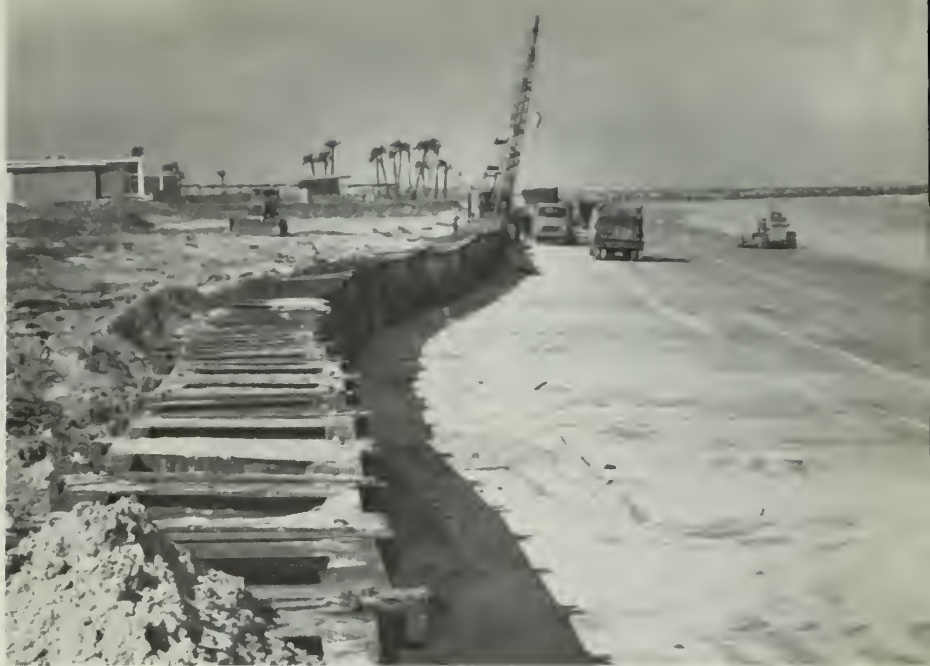
BEACH PARTY —Seabees place pontoons along shore to form barrier. Left : Steelworker cut holes in top of pontoons.
